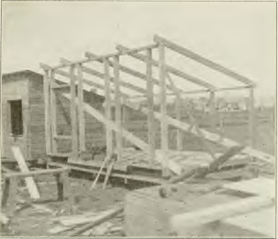
Fig. 17. Portable colony house in process of construction.
